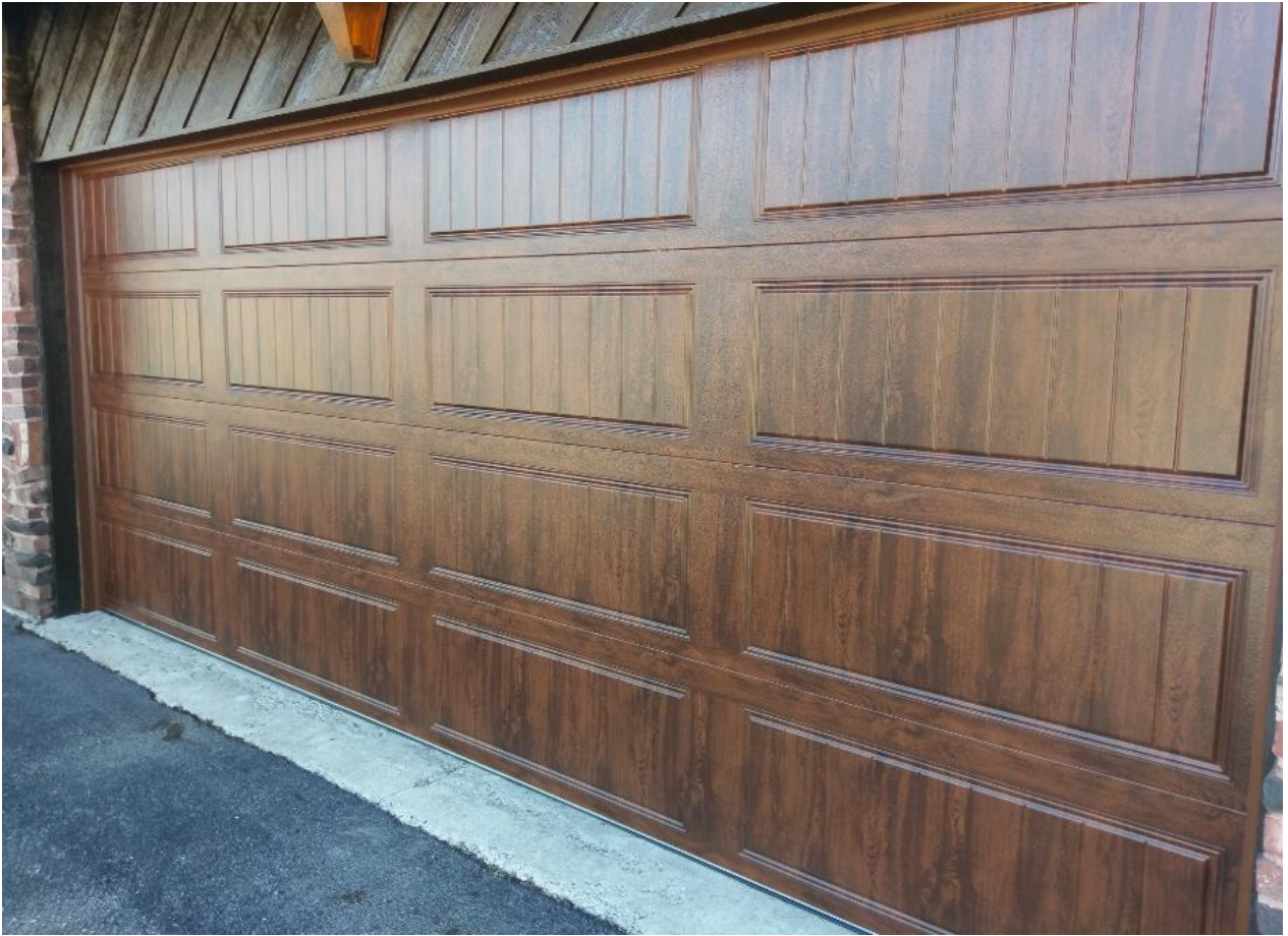
Exhibit K: Steel Overhead Door
